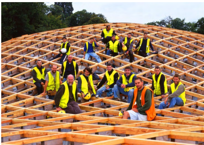
Figure 17 The gridshell construction team
