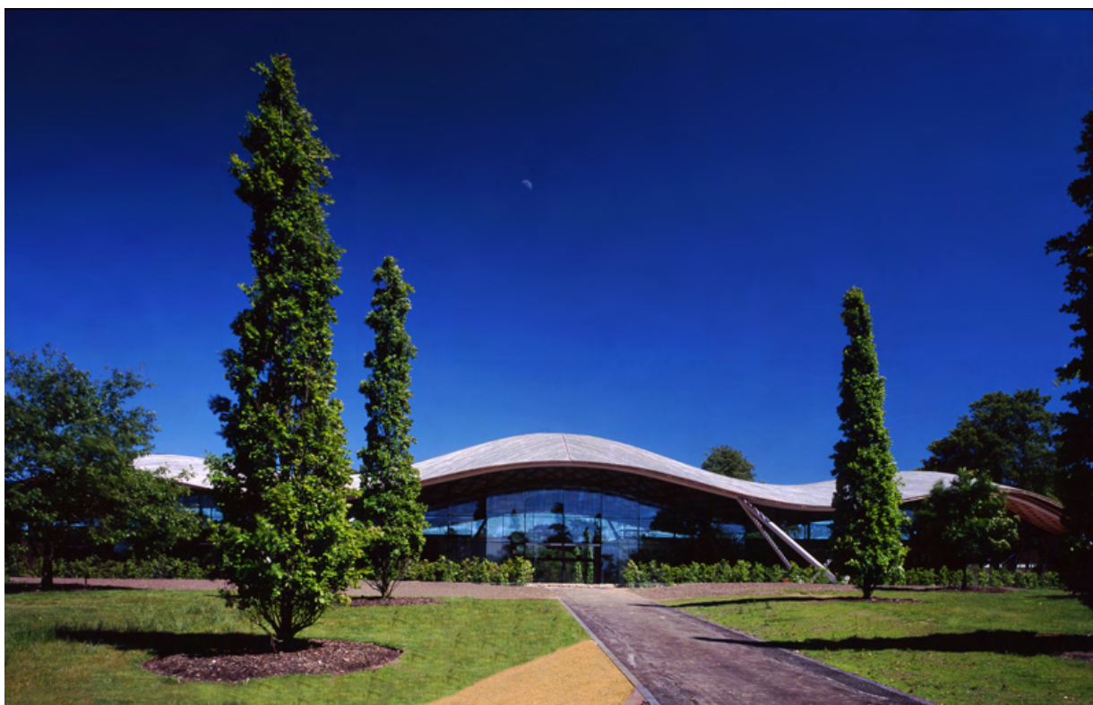
Figure 19 The completed Savill Building
